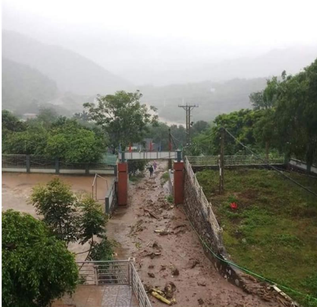
A local road is eroded in Muong Lat District in central Thanh Hoa Province which has been isolated due to heavy downpour and floods over the past days. — VNA/VNS Photo
